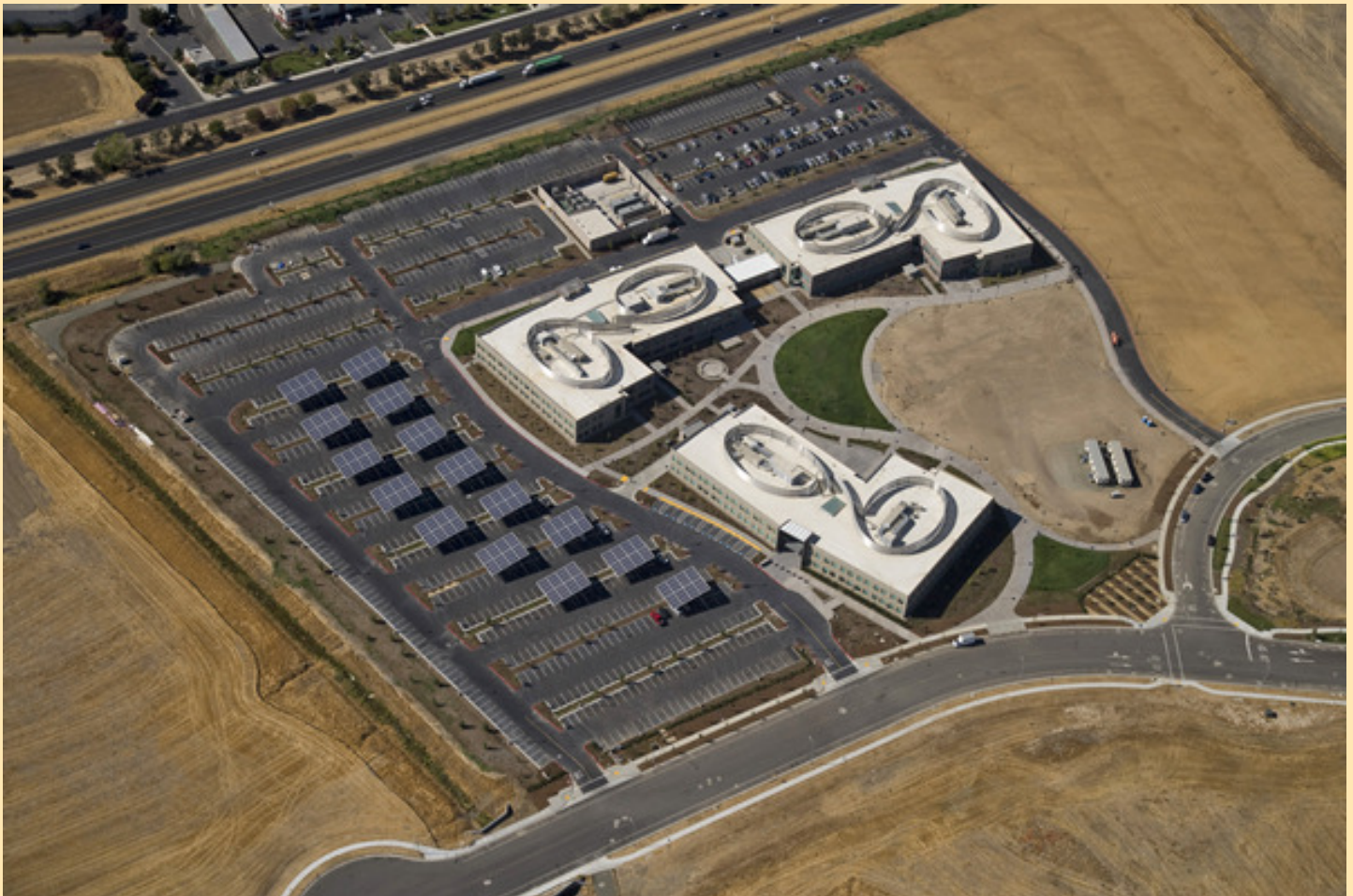
Solar Powered Car Port Structures Installed by Cupertino Electric
