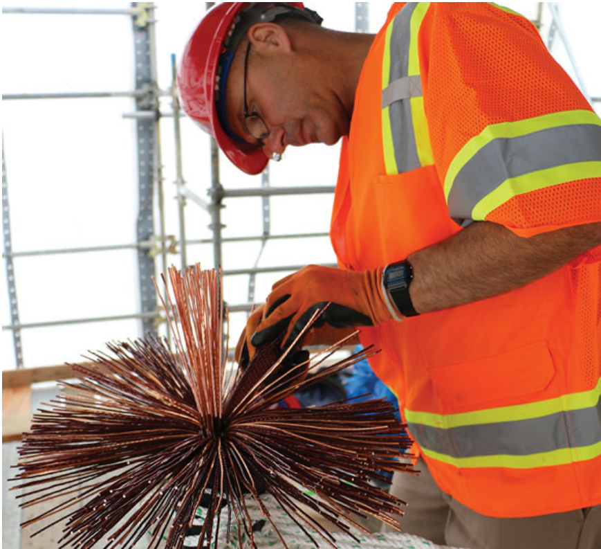
An E-J Electric employee cleans the enamel coating off a power cable in preparation of its termination (Photo courtesy of E-J Electric).
