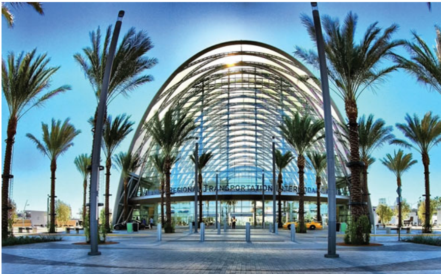
Helix Electric provided the complete electrical infrastructure to power this building, which features more than 1,500 color-changing LED luminaires that illuminate the ETFE roof structure, a distribution system complete with emergency power generation, and uninterruptable power supply system for the protection of critical transportation processes (Photo courtesy of Helix Electric).
