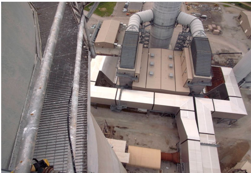
Sachs is performing the balance of the upgrade at Newton Power Station, including all electrical installations (Photo courtesy of Sachs Electric Co.).
