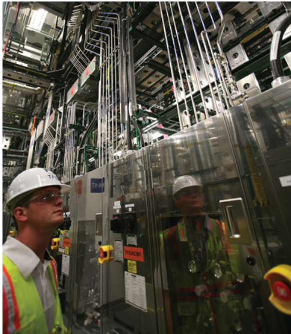
TFS is proud of the dedication and support from its workforce to safely build high-tech projects across the state of New York. Pictured above, a member of the team performs quality checks prior to system turnover (Photo courtesy of Total Facility Solutions).
