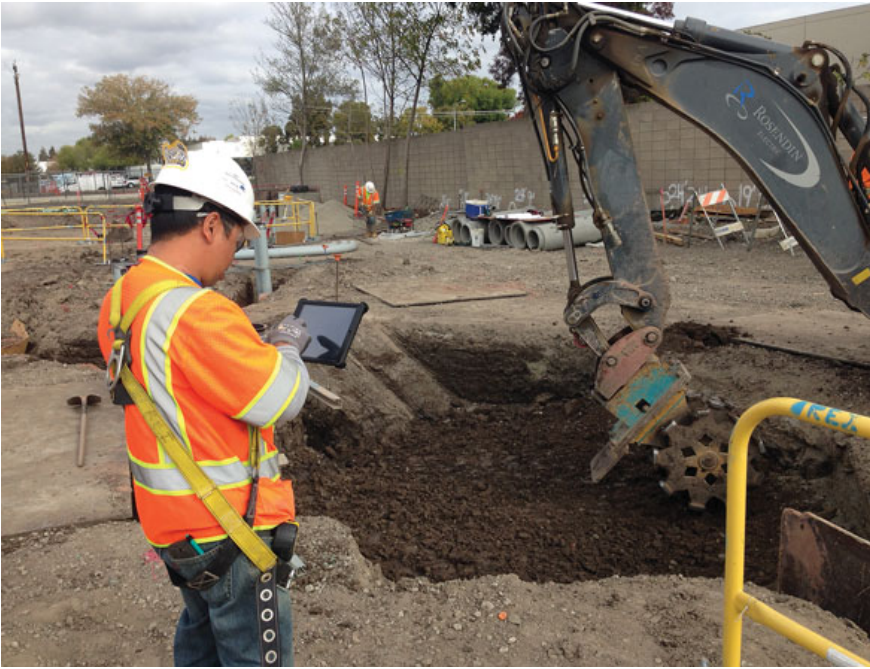
This Rosendin Electric electrician is using mobile technology on the 10-mile BART extension project into Santa Clara Valley. The new line will connect the existing Fremont Station to a new station in Milpitas and terminate at the first San Jose BART Station, Berryessa (Photo courtesy of Rosendin Electric).
