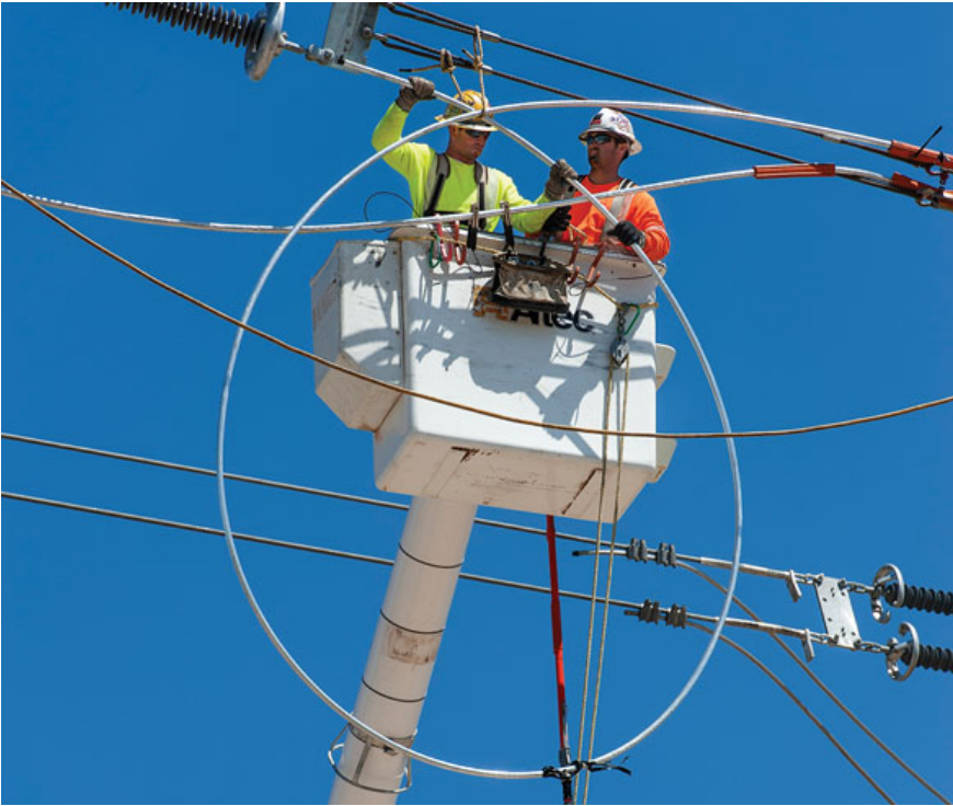
Quanta Services linemen work on a transmission line in Texas (Photo courtesy of Quanta Services).
