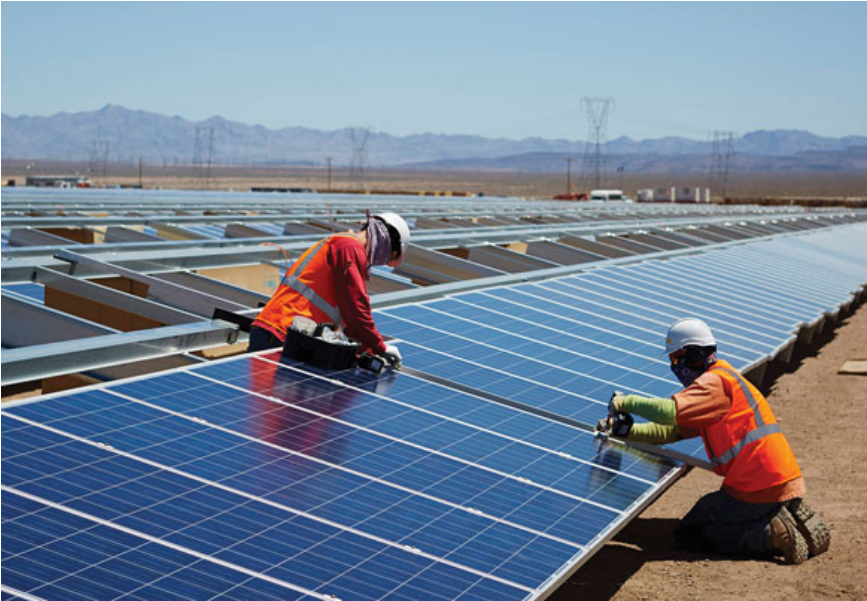
Cupertino Electric employees installed a large number of solar panels at the Copper Mountain Solar 3 project in Nevada (photo courtesy of Cupertino Electric).
