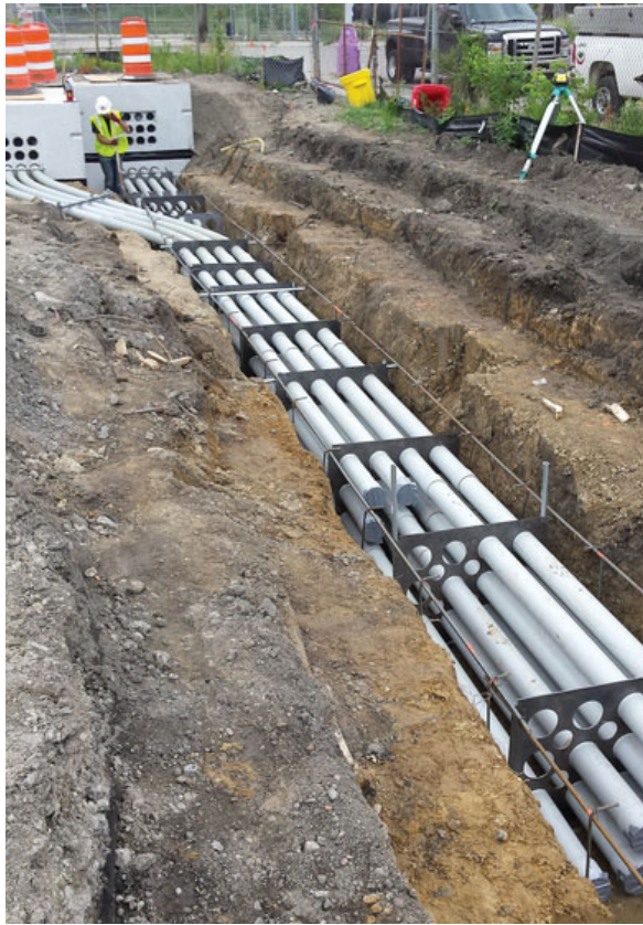
Motor City Electric worked on the Quicken Loans Technology Center, a 66,000-square-foot data center and office complex in Detroit. MCE's fab shop produced the conduit spacers for the duct bank, which helped cut costs and increase productivity (Photo courtesy of Motor City Electric Co.).
