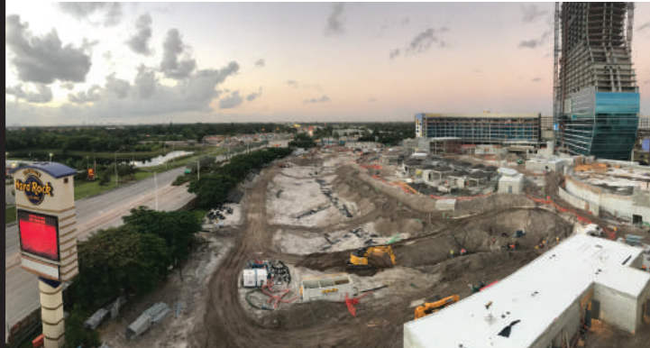
Brightview Landscapes (No. 33) is building a 10-acre pool complex that includes a lagoon pool, “Bora Bora” pools, a river pool, a VIP-suite pool and multiple waterfalls at the Hard Rock Hotel & Casino in Hollywood, Fla. ■
