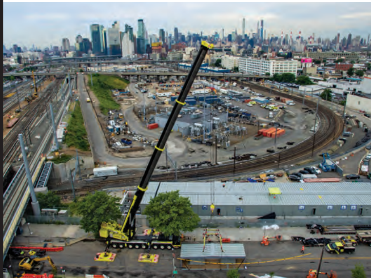
E-J Electric Installation Co. ( No. 36 ) installs one of the last segments of the largest prefabricated traction power substation in the U.S. for Long Island Railroad's East Side Access Program. The building stretches 250 ft.
